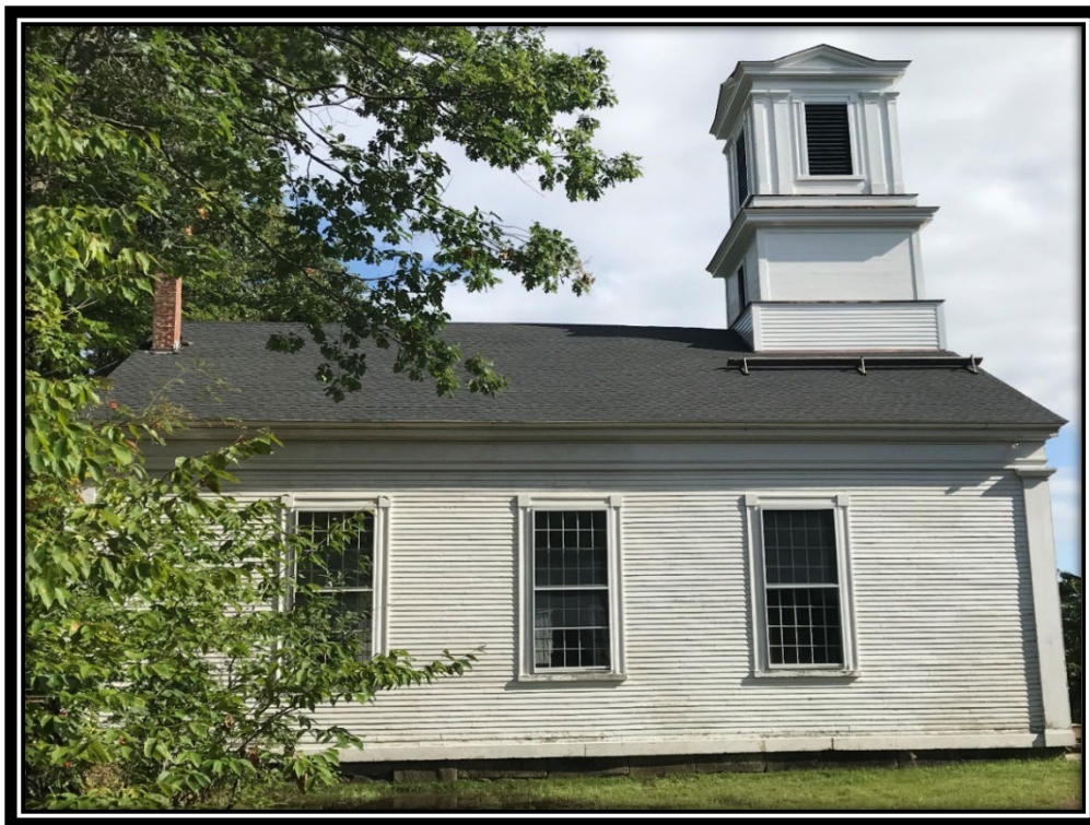
Structure is now secure – waiting for spring 2022 for mason
