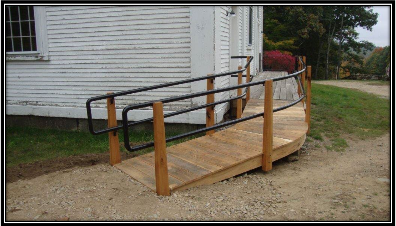
New ADA ramp up to code
