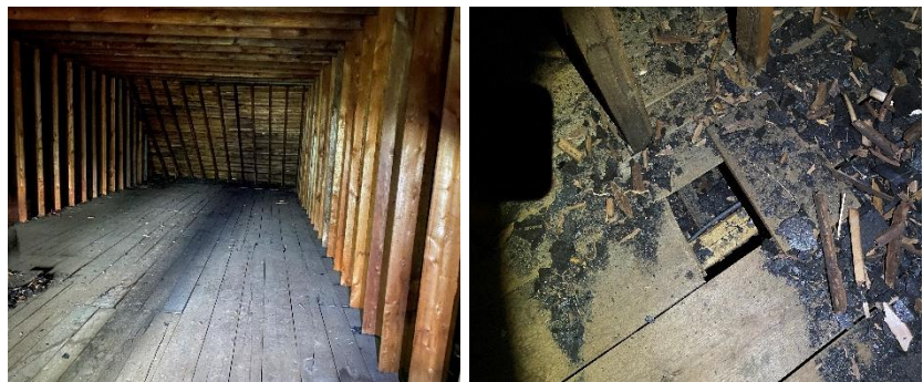
Figure 1. Uninsulated attic proper
