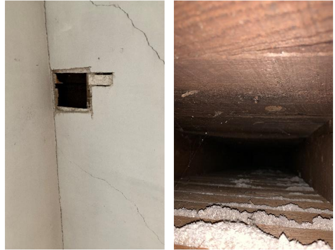
Figure 2. Uninsulated wall cavity
