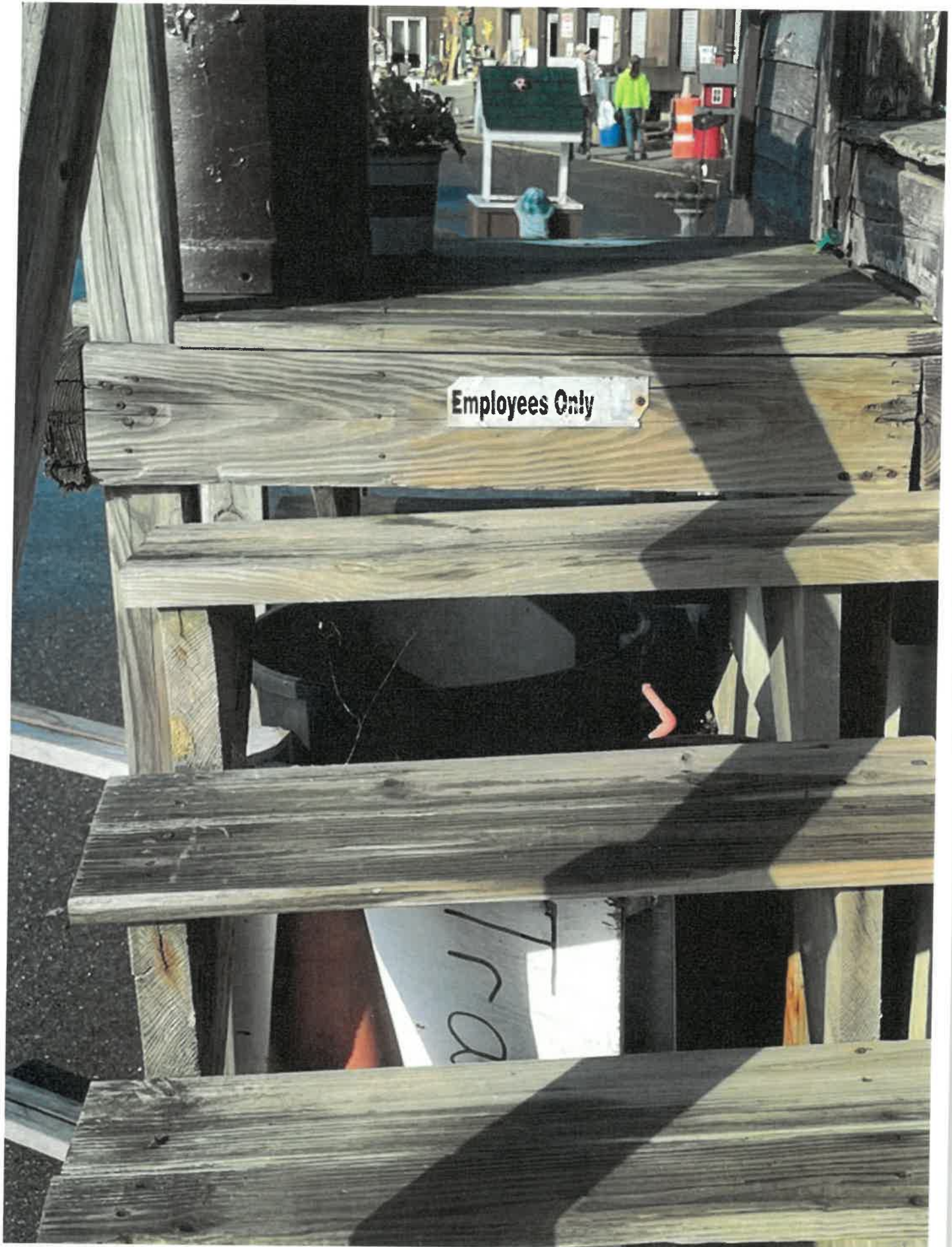
Control room entrance
