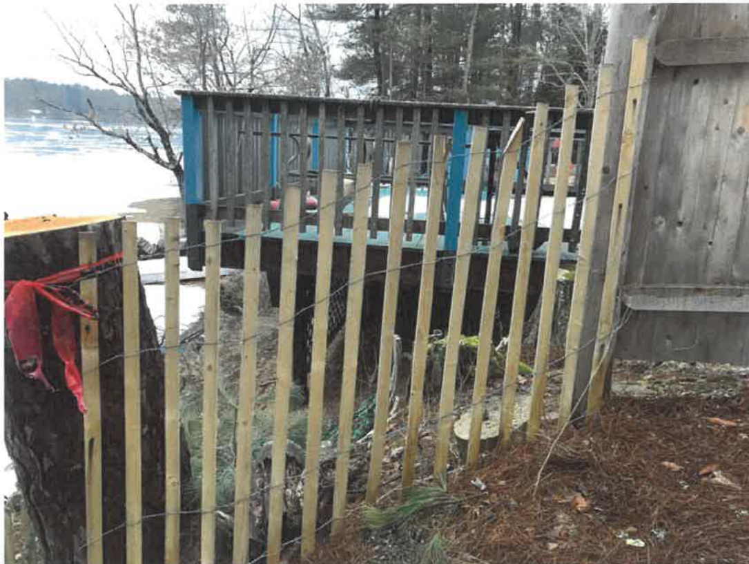
Photo Point 8: 2-28-2024 – a view over the northerly property line showing the deck on the abutting property at 7 Bacon Way (Tax Parcel 110-007).
