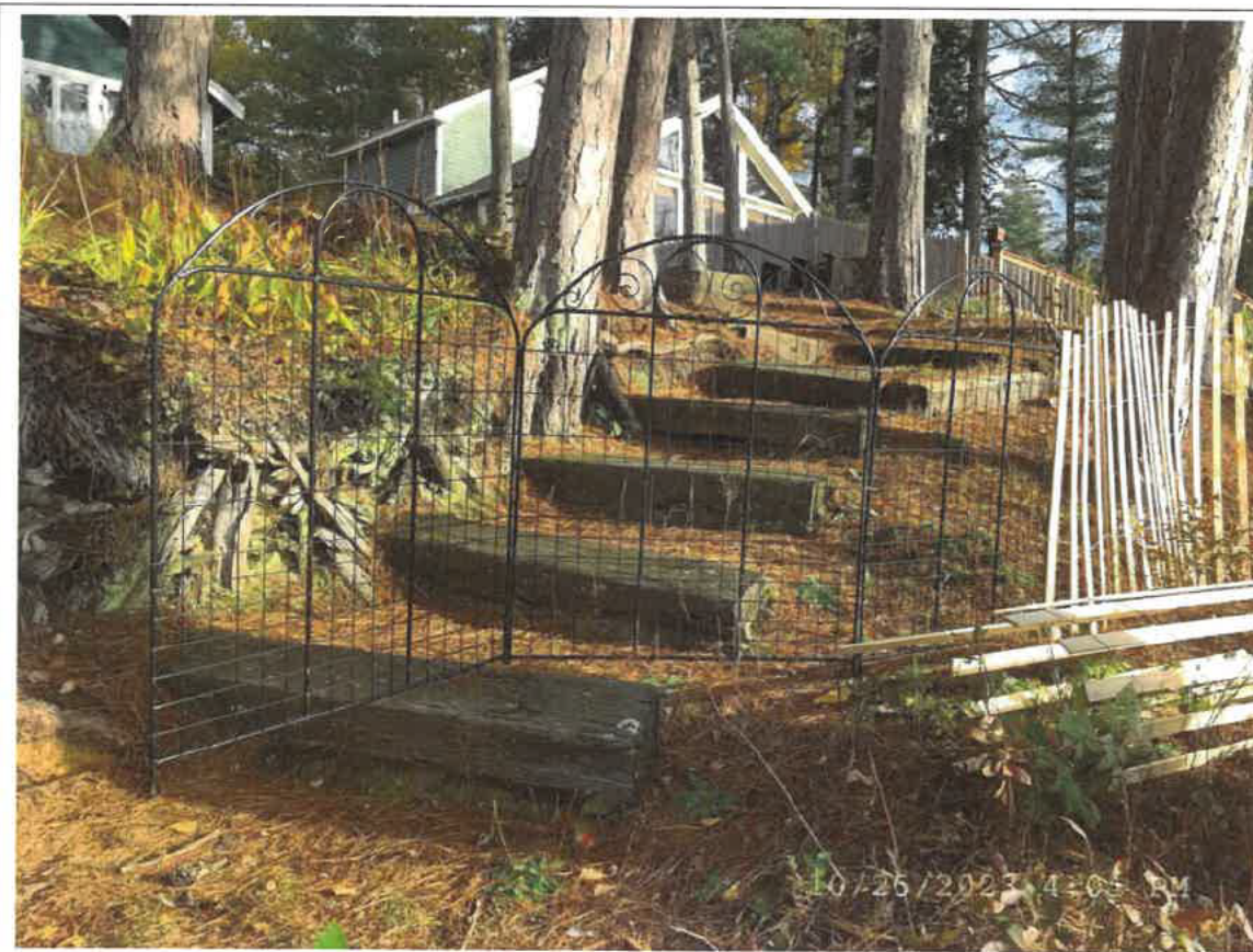
Photo Point 6: 10-25-2023 Southeasterly view showing existing landscape tie steps. These steps are proposed to be left in place with the space between steps planted with low-bush blueberry plants. Note: some tree cutting has occurred since this photo – all stumps are in place and the point scores are met per grid (See Sheet 6 of Plan Set).
