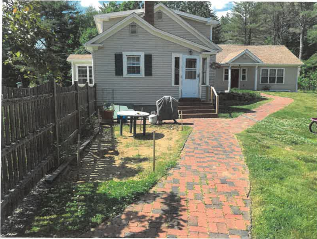
6-25-2022: Northerly view taken from garage. The proposed pergola/patio is between the fence and brick walkway. The grade stakes are approximate locations of the vertical posts.
